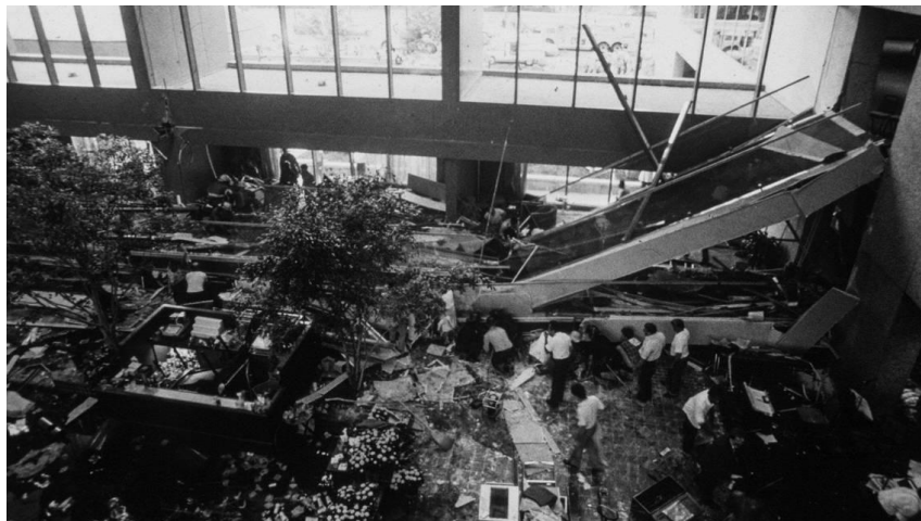
Figure 1.1 Wreckage of the collapsed Hyatt Regency Hotel in Kansas City.
