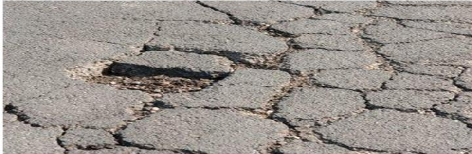
Fig.4. Pot holes due to the frost heaves
