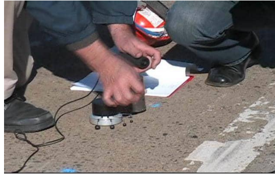
Fig: Testing of Concrete Member
