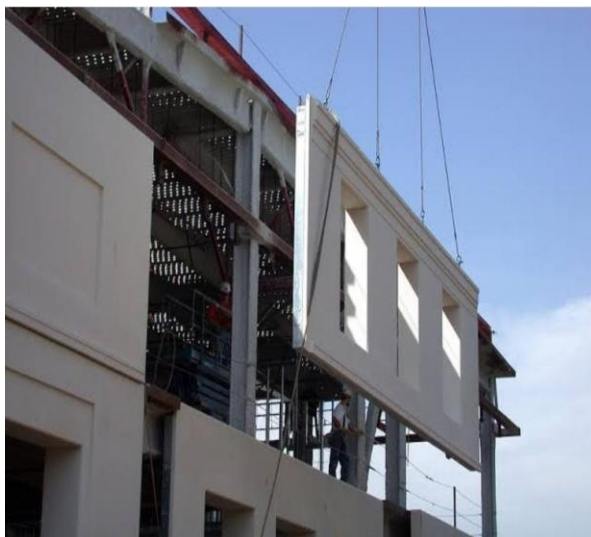
Figure 1.1: Construction stage of a precast wall panelled building
