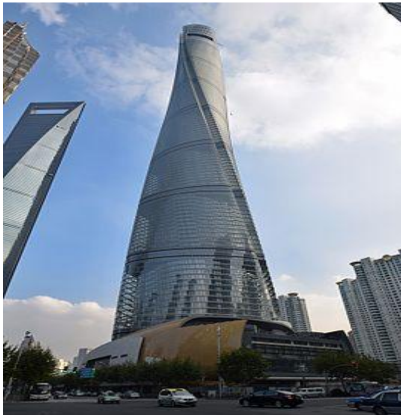
Figure 1: The Shanghai Tower
