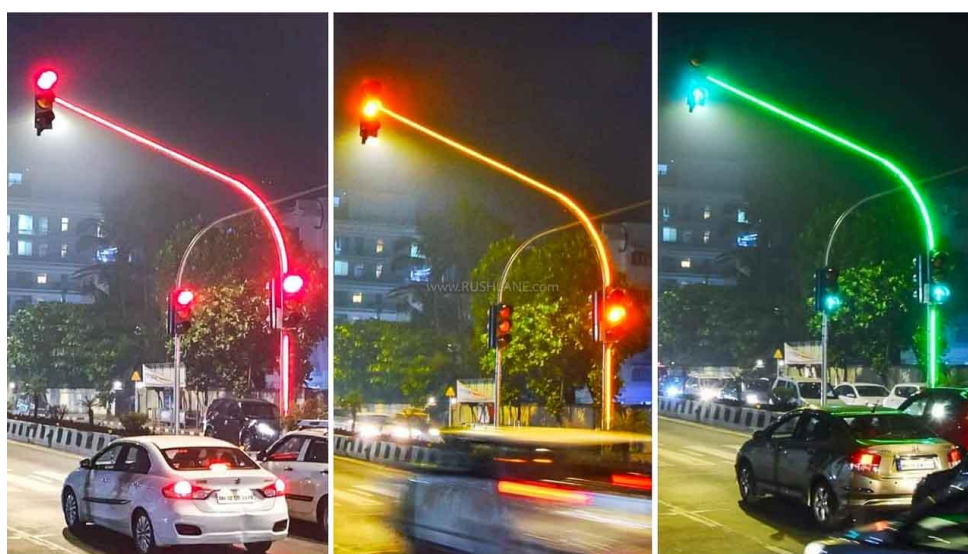
FIG:- IMPROVEMENT OF STREET LIGHT IDEAS
