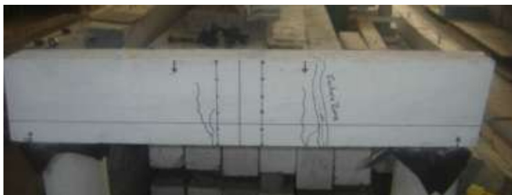
Figure 8 Failure Mode of Beam (B3)
