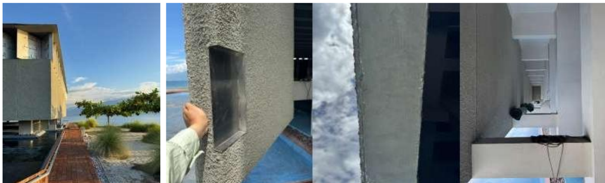
Figure 10: Wall Elements of the Nurul Yaqin Mosque (Exterior View and Interior View)
