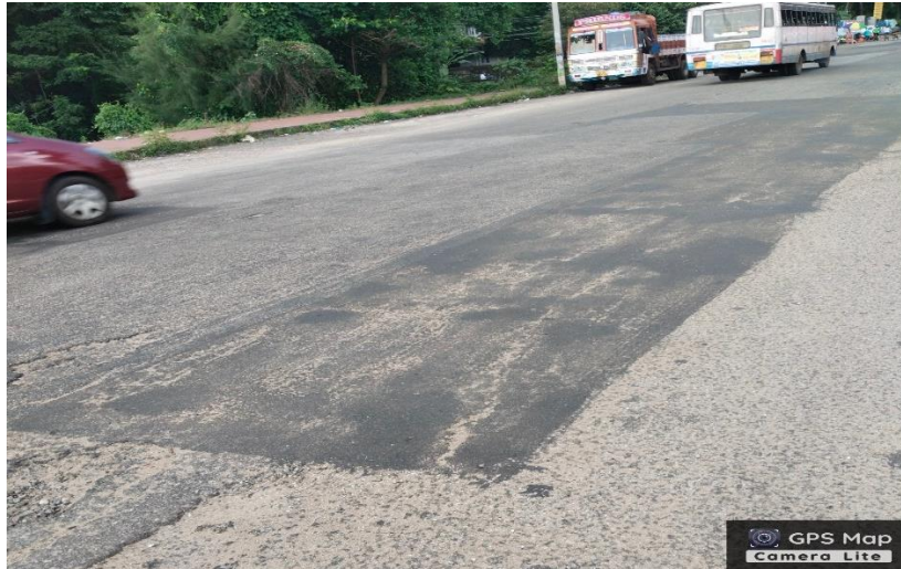
Figure 1: Road section with patch works
