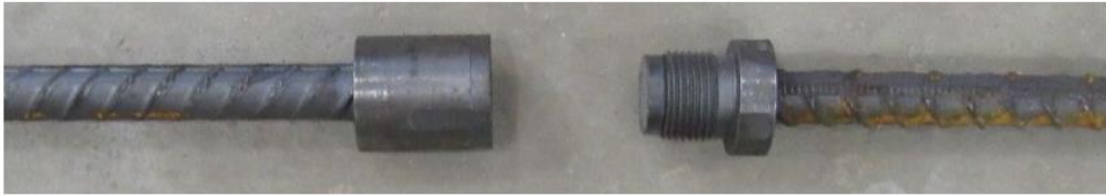
Figure 1.2 Header type mechanical joint
