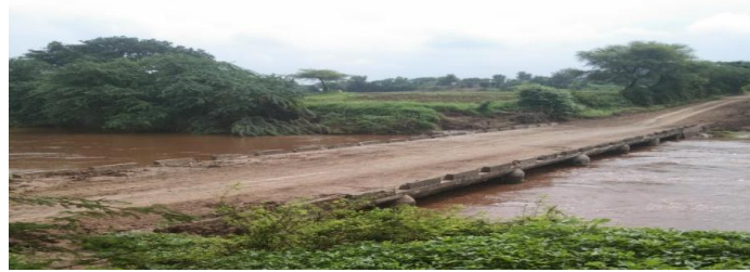
Figure 1: High Level Causeway at Naved-Darapur Road
