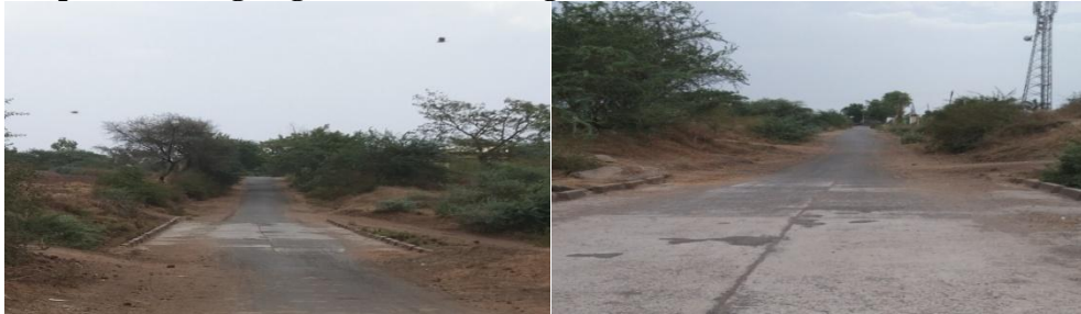
Figure 7: High Slope Road Connecting the Bridge
