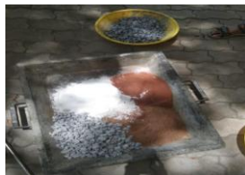
Dry mix of geopolymer concrete
