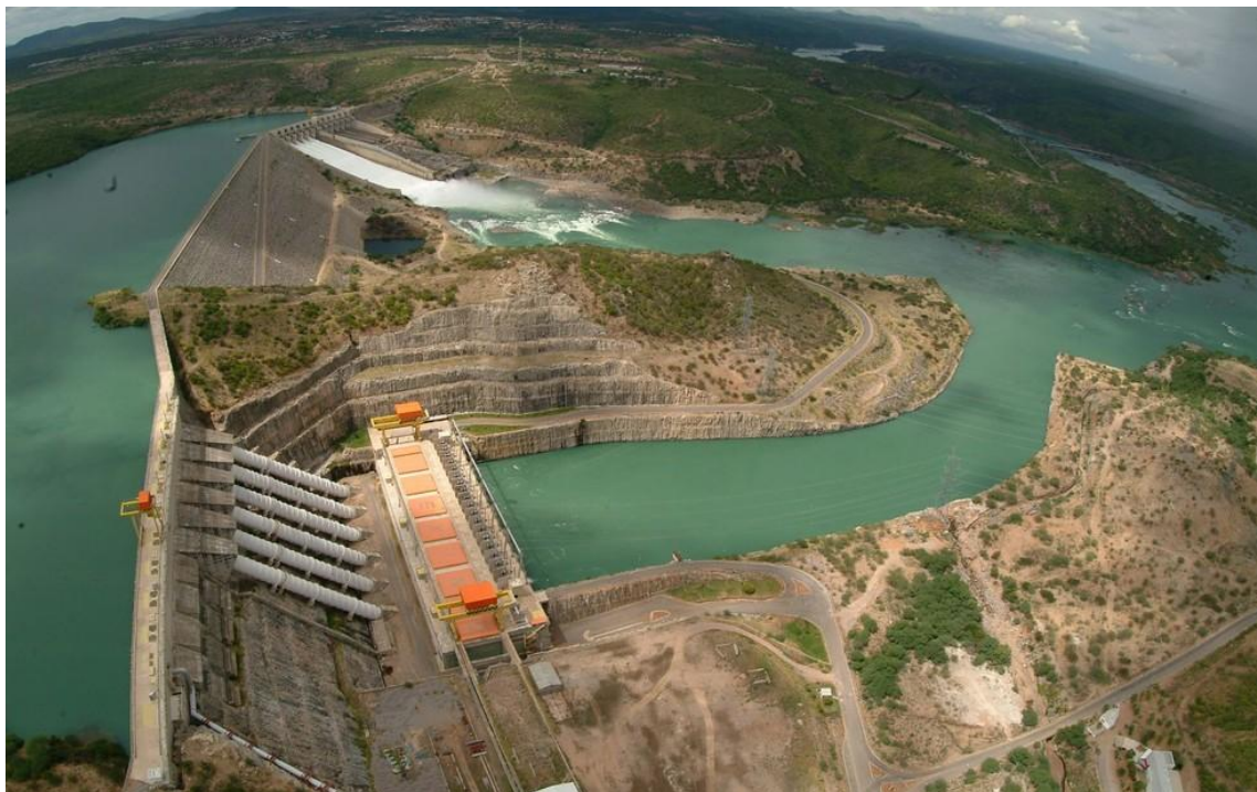
Figure 2: Object of study – Xingó HPP [Source: PORTAL G1 SERGIPE. Xingó Hydroelectric Power Plant expands flow to 2.000 cubic meters starting this Saturday.
