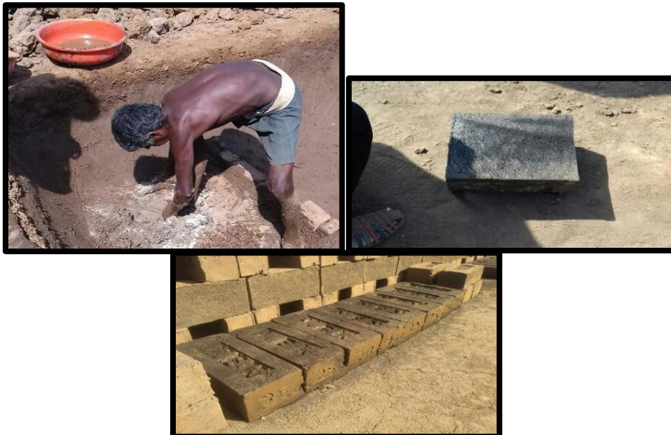
Sample Image of Making and placing of bricks
