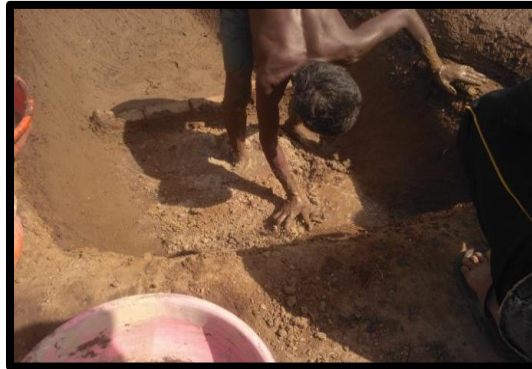
Figure: 2.8: Material mix at site
