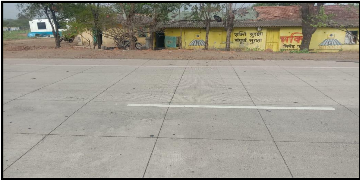
Figure 4.1: white topping road after finishing
