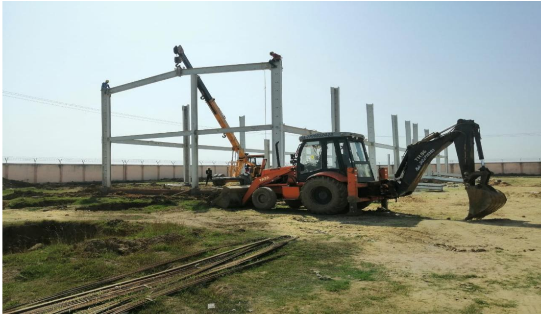
STAGE 8 ROOF BEAM ERECTION WORK- After complete the joist beam installation work then we start the roof beam erection work.
