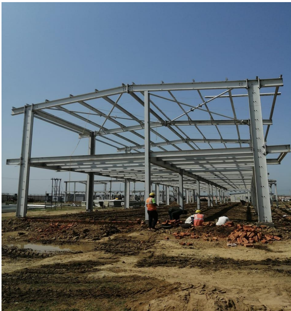
STAGE 8 ROOF BEAM ERECTION WORK- After complete the joist beam installation work then we start the roof beam erection work.
