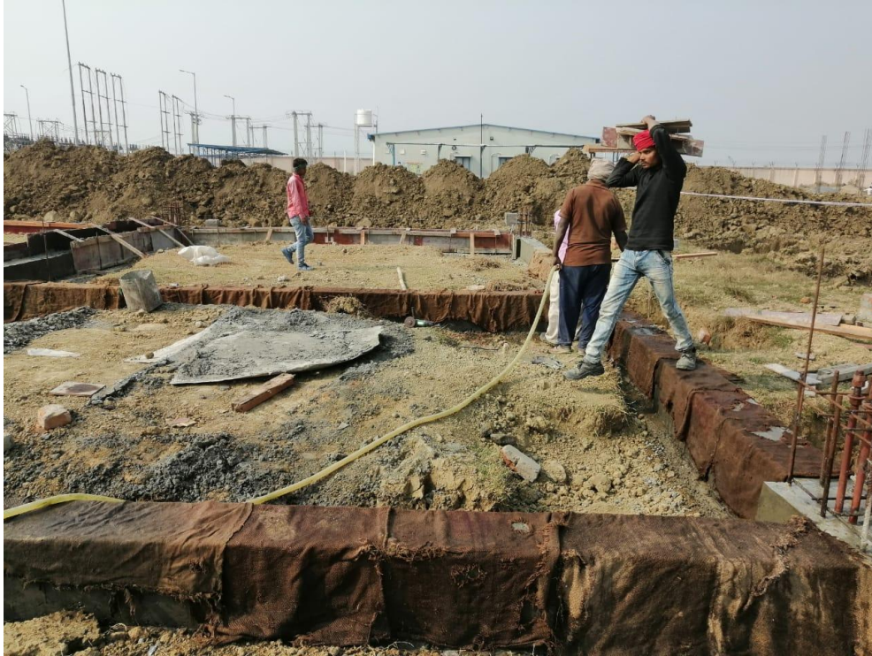
STAGE 5 BRICKWORK -making full brickwork (230 mm) throughout the outer grid of the building at the height of 400-500 mm and also casting column at the height of 600 mm. after the brickwork backfilling the building at the height of 600 mm.
