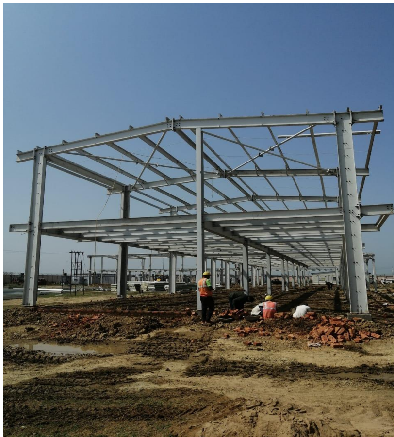
STAGE 5 BRICKWORK -making full brickwork (230 mm) throughout the outer grid of the building at the height of 400-500 mm and also casting column at the height of 600 mm. after the brickwork backfilling the building at the height of 600 mm.
