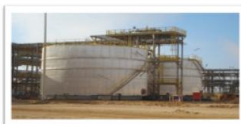
Figure 2: Fixed pressure type tank
