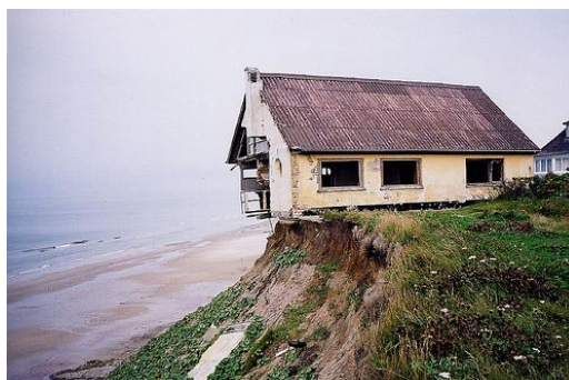
Figure1: Photographs of landslides
