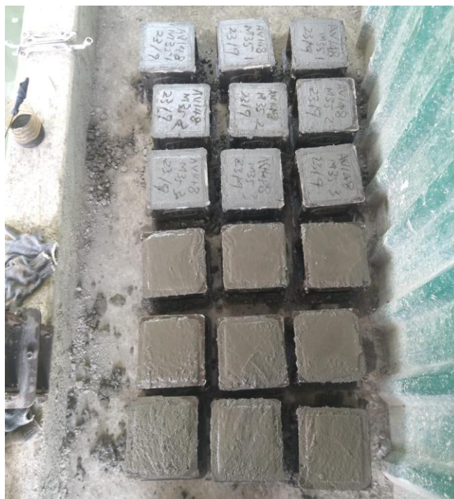
Fig 5.9 Casting of aloe vera concrete in cubes
