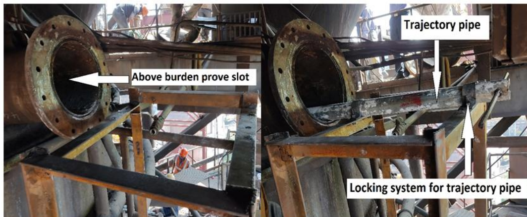
Figure-5: Chalk line probe fixing
